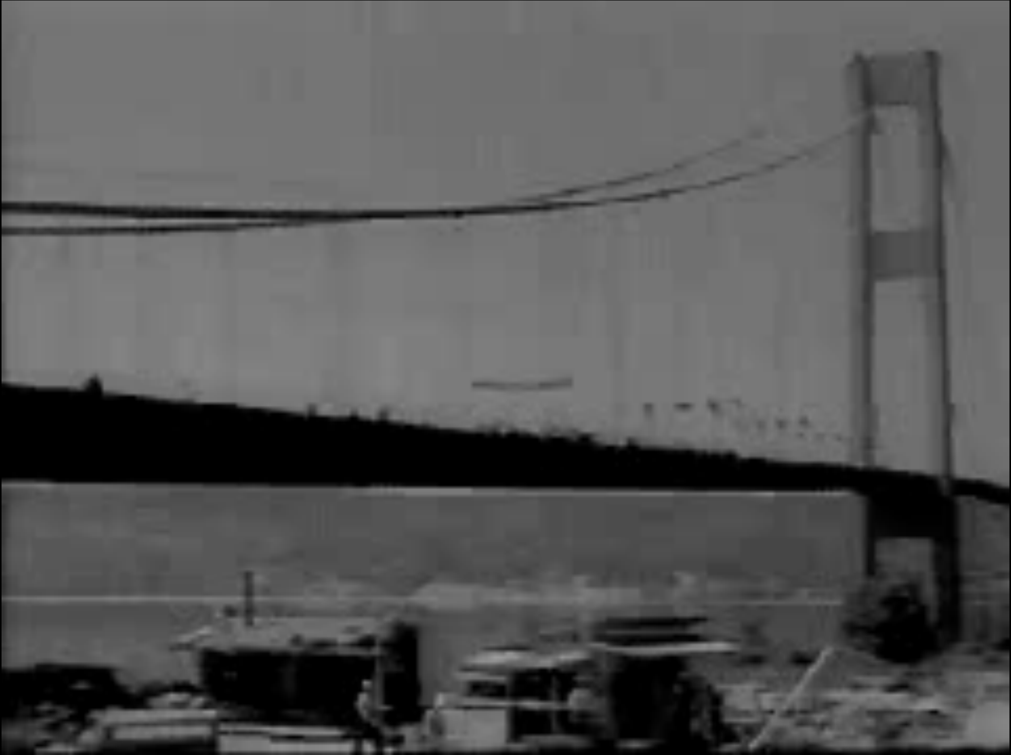
1940 collapse of the Tacoma Narrows Bridge
